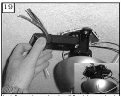
Install remote receiver by sliding into opening in the Mounting bracket. Make sure that the dip switches on the Transmitter and the Receiver are set to the same position. See Fig 34 for remote operation
